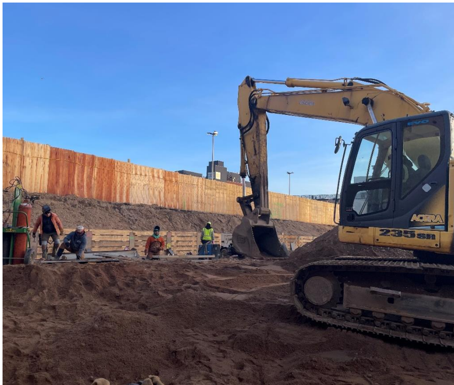
Photo 2: View of contractor welding H piles in Lot 14, facing north-northeast.
