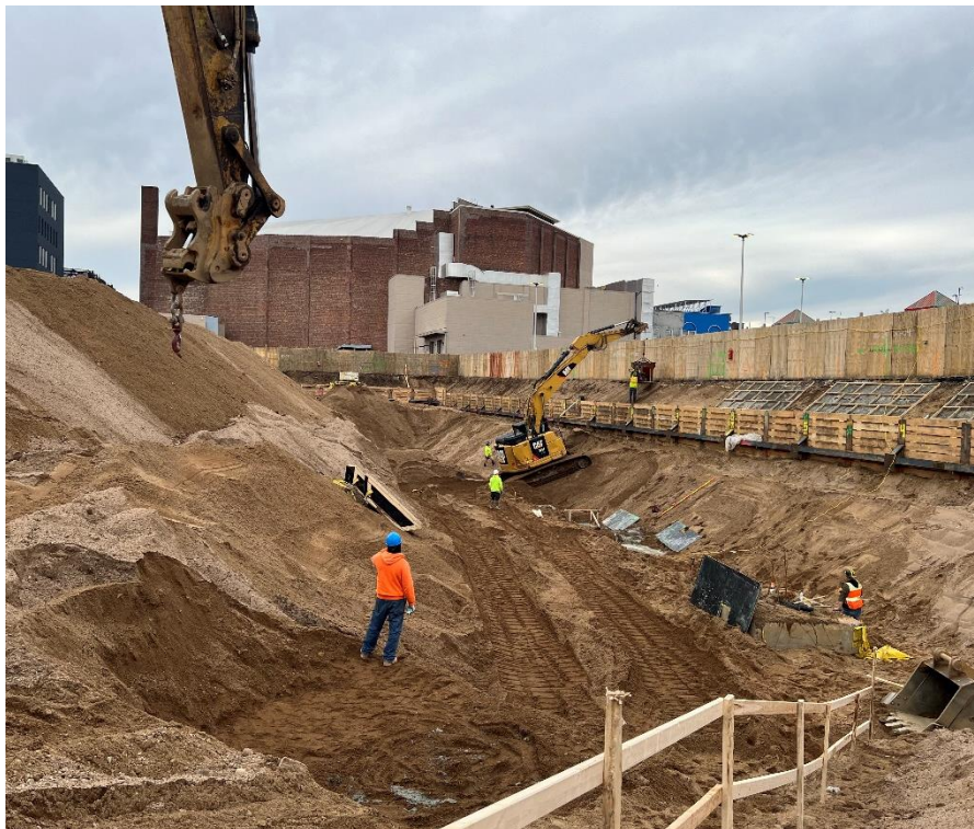
Photo 2: View of SOE work from Lot 14, facing northwest.
