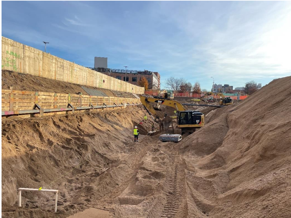
Photo 2: View of SOE work from Lot 14, facing east.
