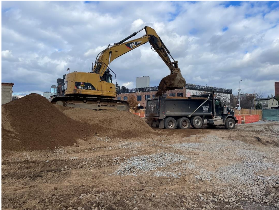
Photo 2: View of contractor loading soil on Lot 14, facing northeast.
