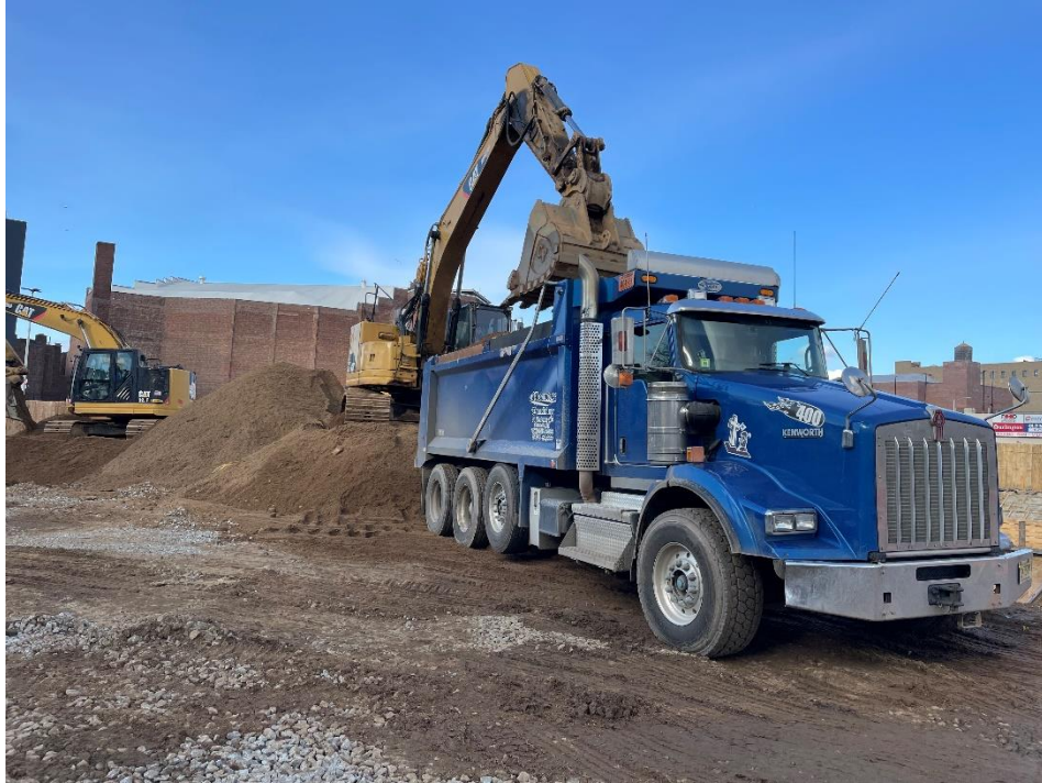
Photo 1: View of contractor loading soil on Lot 14, facing northwest.
