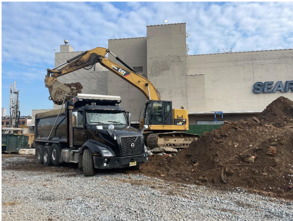
Photo 2: View of contractor loading soil on Lot 14, facing east.
