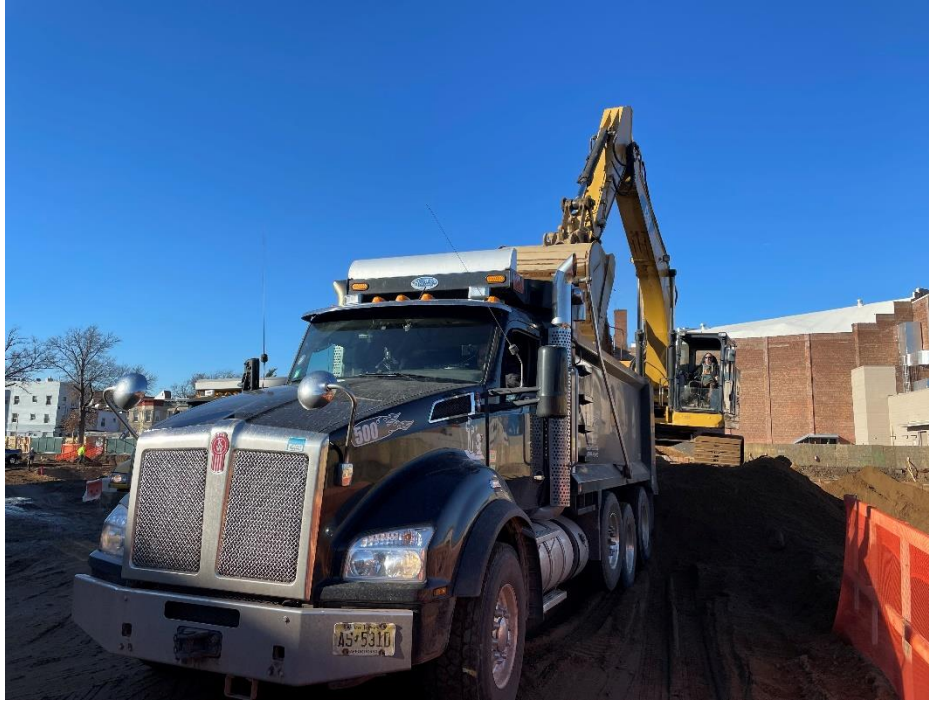
Photo 1: View of contractor loading soil on Lot 14, facing west.
