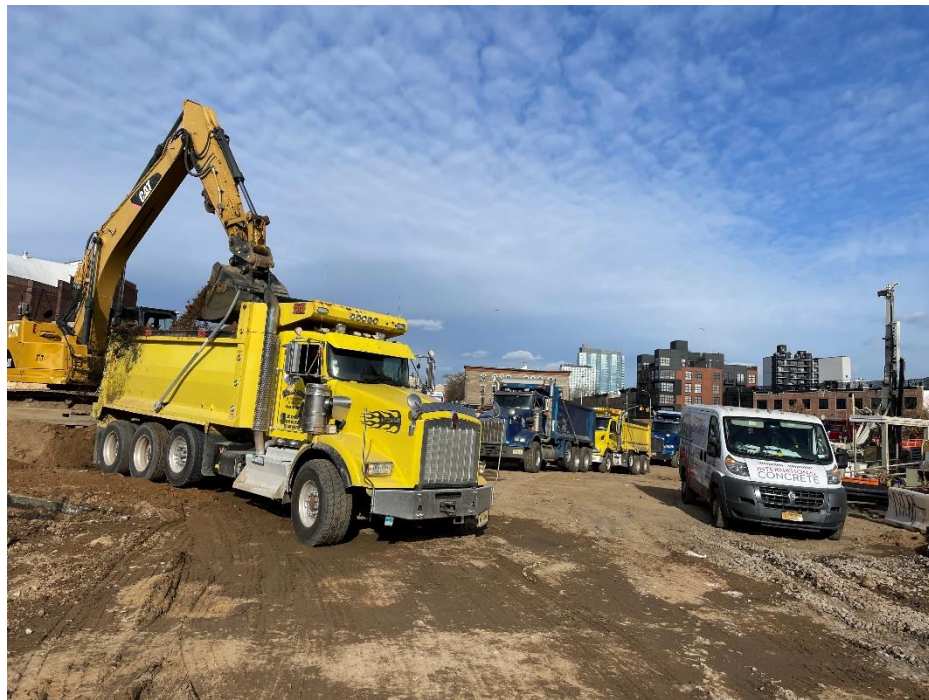
Photo 2: View of contractor loading soil on Lot 14, facing north.
