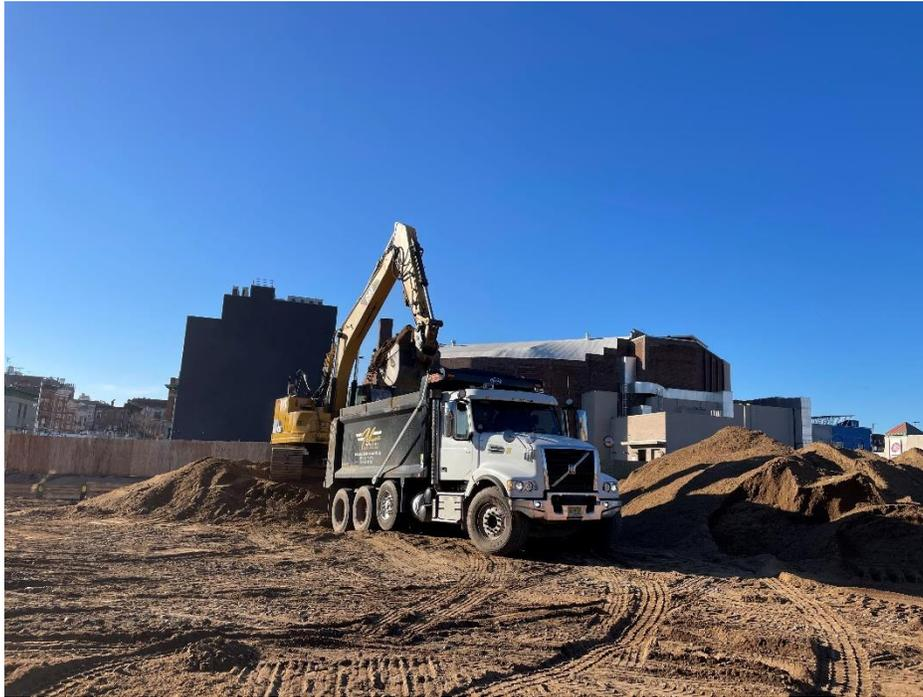
*Photo 1: View of contractor loading soil for off-site disposal on Lot 14, facing west.*
