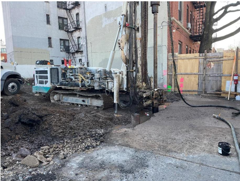
*Photo 2: View of contractor installing piles on Lot 53, facing south-southeast.*
