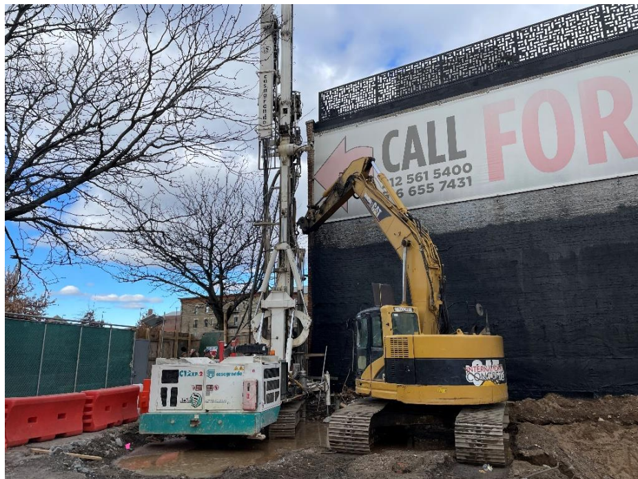
Photo 2: View of contractor installing piles in Lot 53, facing north-northwest.
