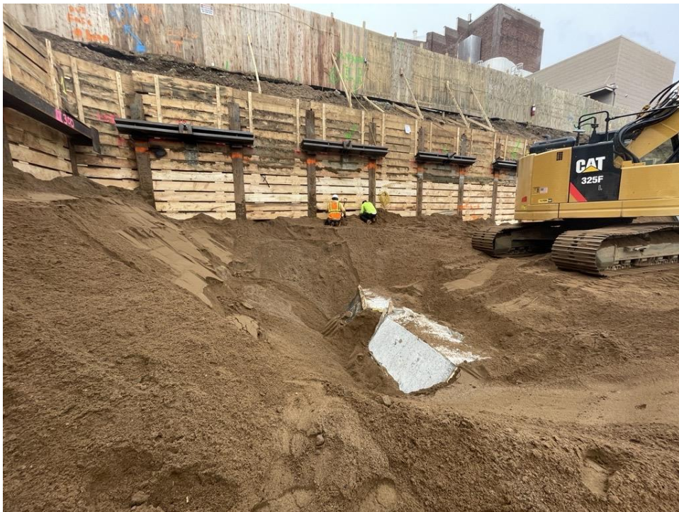
Photo 2: View of contractor SOE installation in Lot 14, facing north-north east.
