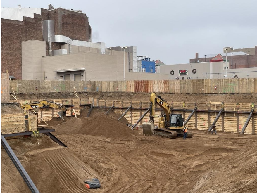
Photo 1: View of SOE activities on Lot 14, facing north-northwest.
