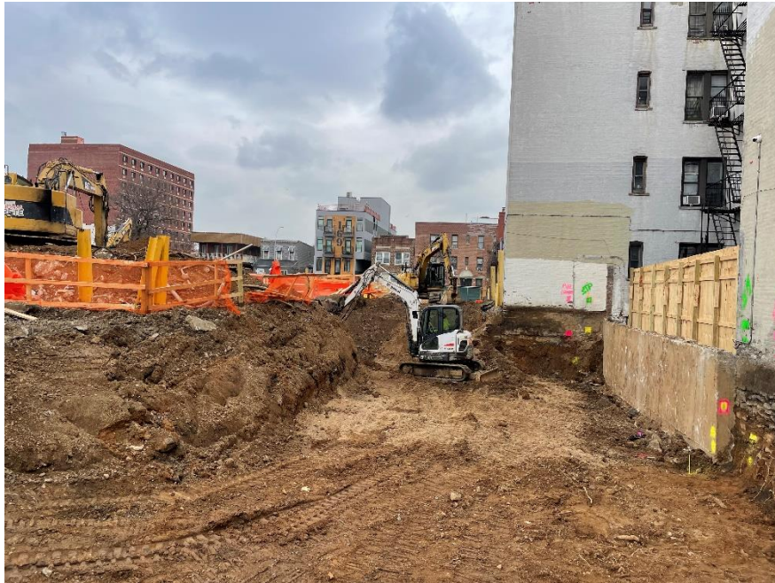
Photo 2: View of SOE activities in Lot 53, facing southeast.
