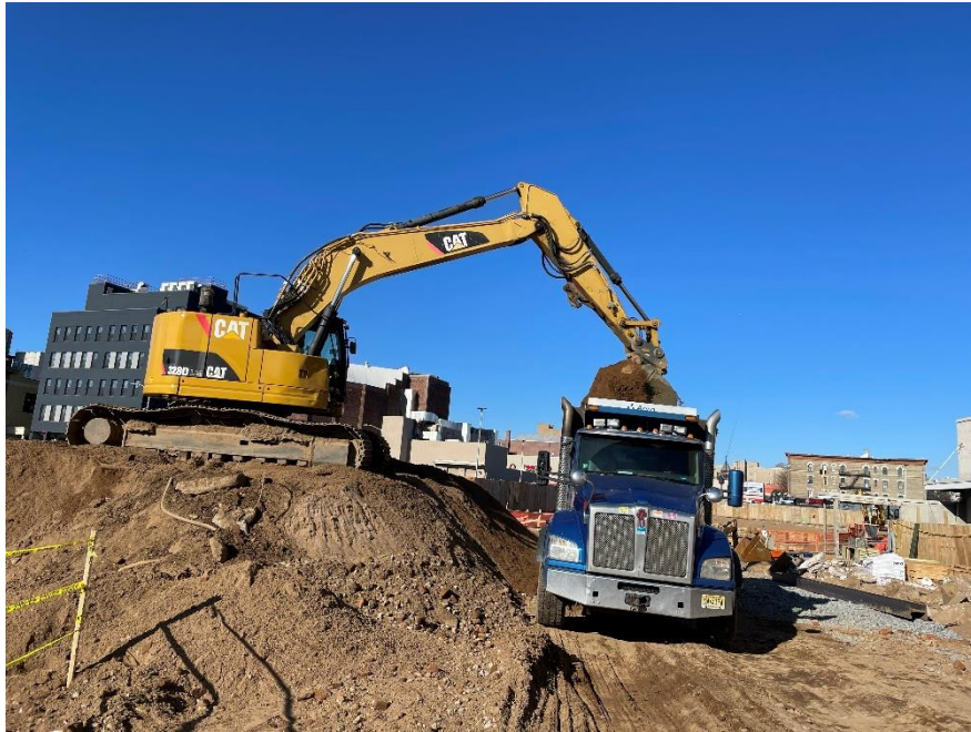
Photo 1: View of soil loading for disposal on Lot 14, facing north.
