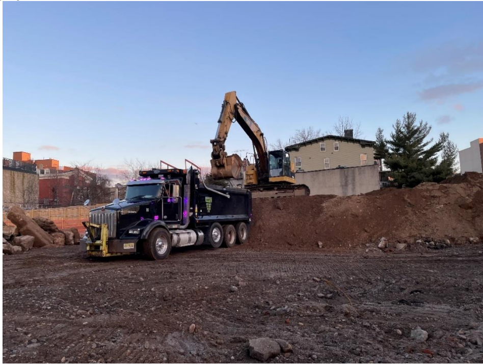
Photo 1: View of soil loading for disposal on Lot 53, facing north.
