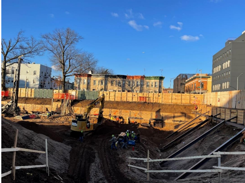
Photo 2: View of SOE activities in Lot 14, facing west-southwest.
