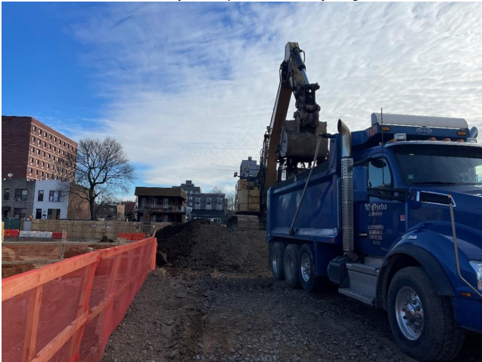
Photo 2: View of soil stockpile in Lot 53, facing east.
