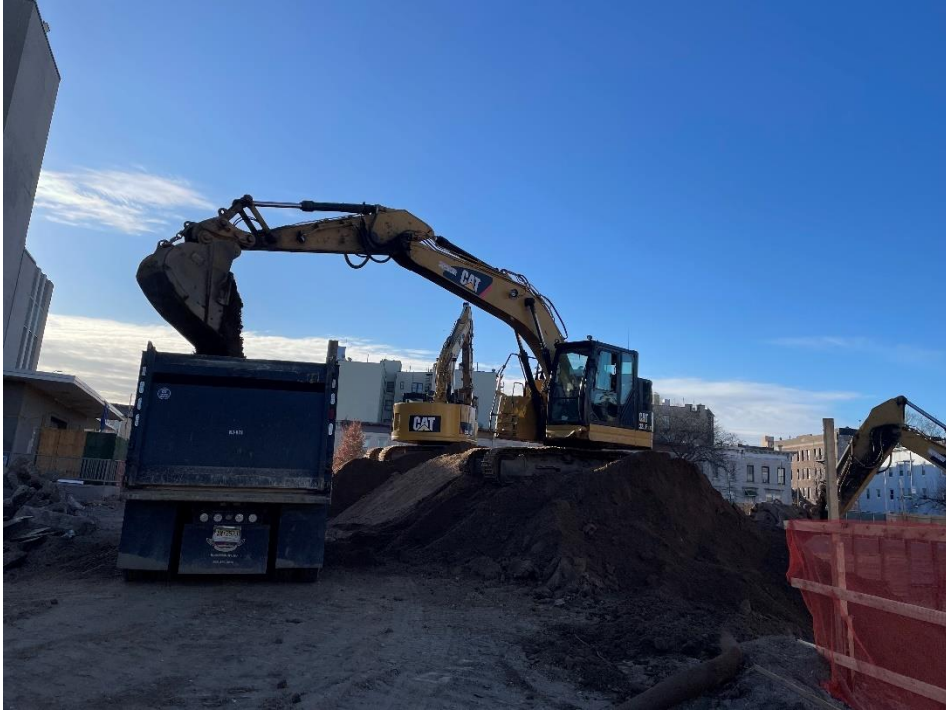
Photo 1: View of soil disposal in Lot 14, facing south.
