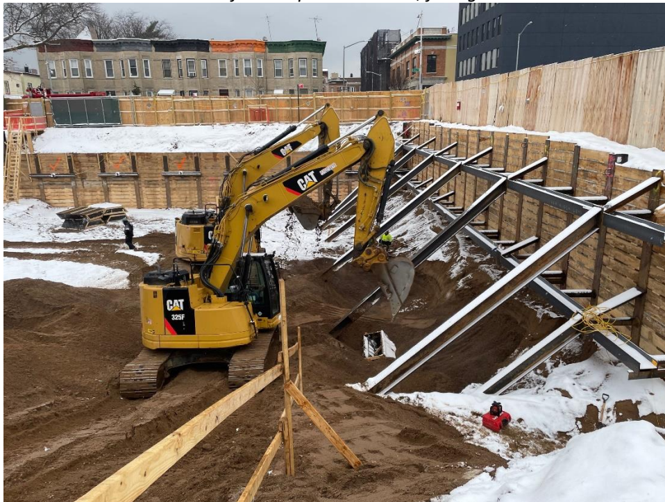
Photo 2: View of SOE Installation in Lot 14, facing west.
