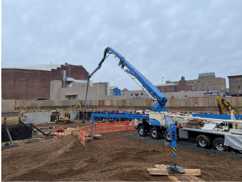
Photo 1: View of contractor pouring concrete on Lot 14, facing northwest.
