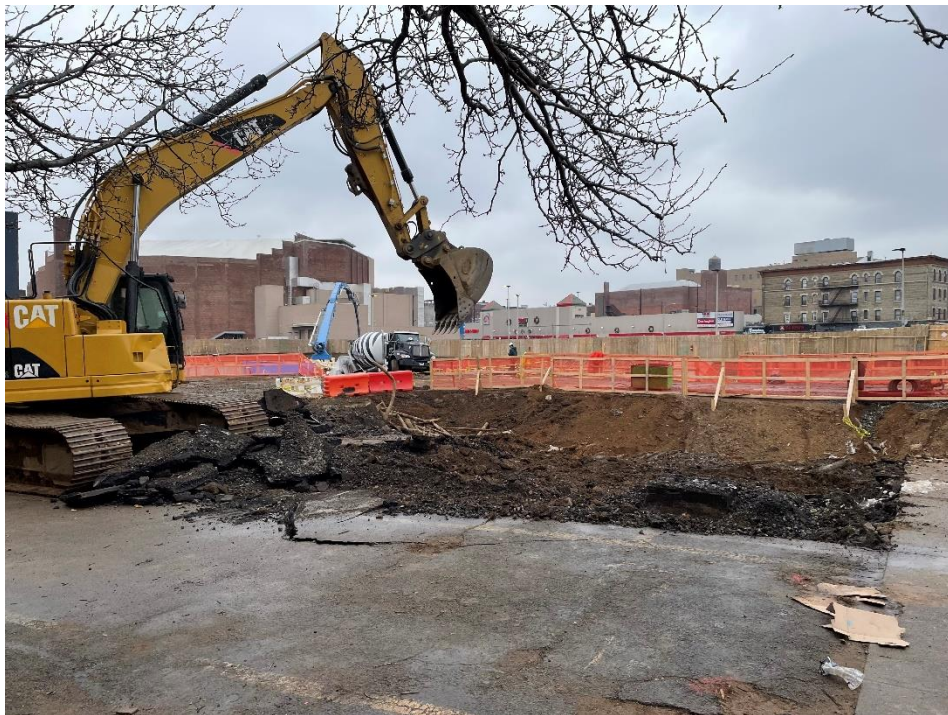
Photo 2: View of contractor removing asphalt in Lot 14, facing north.
