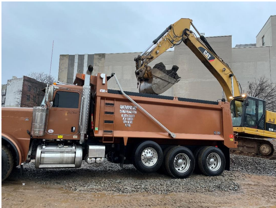
Photo 2: View of contractor loading asphalt in Lot 14, facing south.
