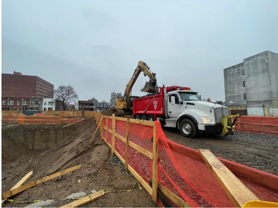
Photo 1: View of contractor loading soil on Lot 53, facing east.
