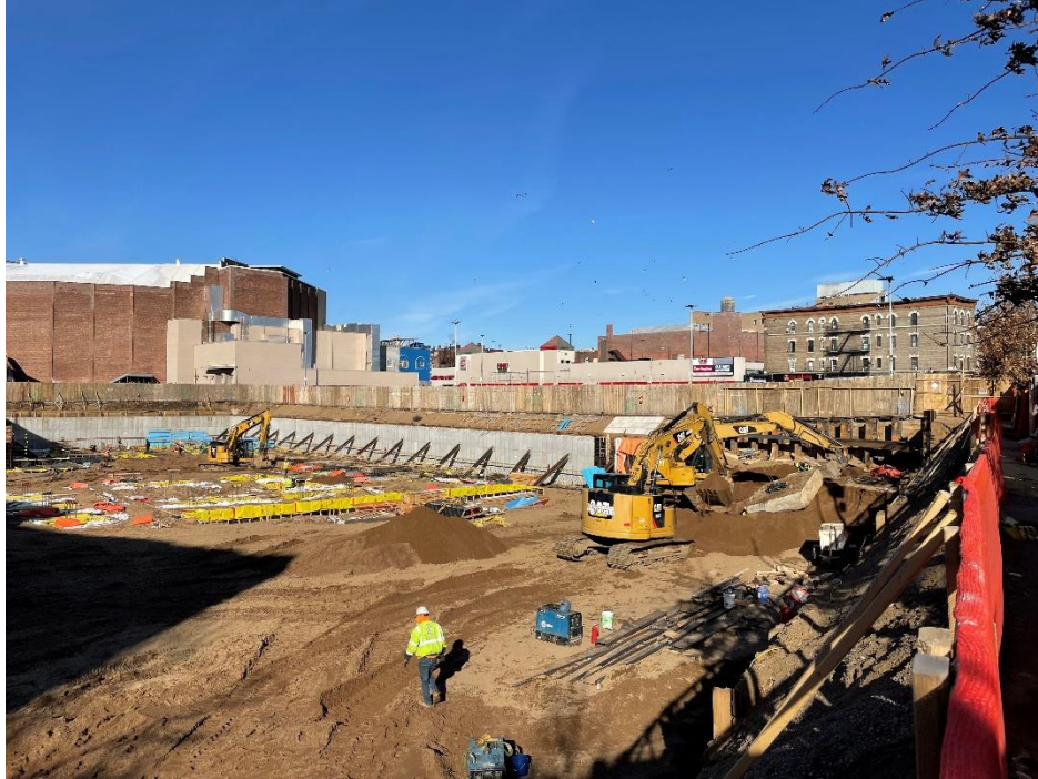
Photo 1: View of site conditions in Lot 14, facing north.
