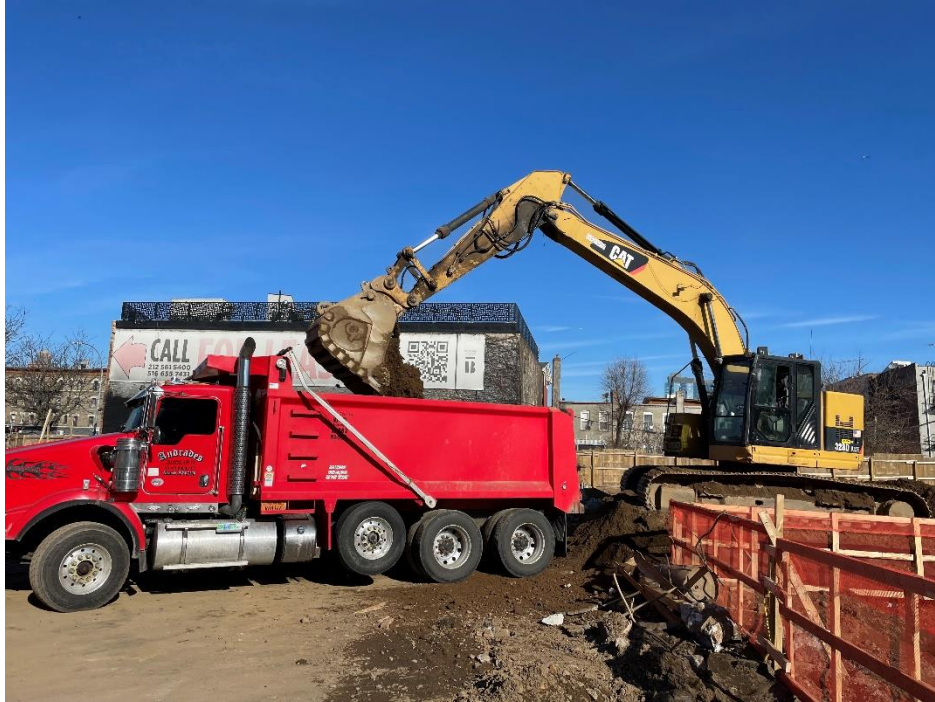
Photo 3: View of contractor loading soil on Lot 53, facing north.
