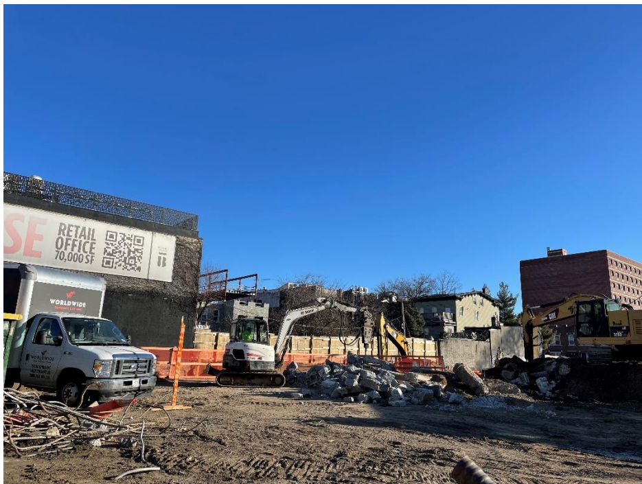
Photo 4: View of contractor breaking C&D on lot 53, facing northeast.
