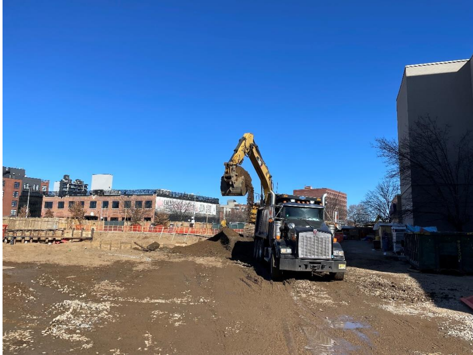
Photo 1: View of contractor loading soil in Lot 14, facing east.
