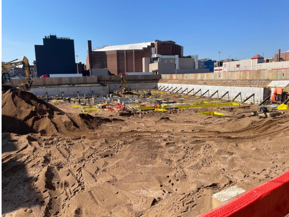
Photo 1: View of soil conditions Lot 14, facing south.
