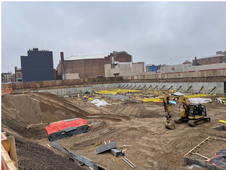
Photo 2: View of site conditions in Lot 14, facing northwest.
