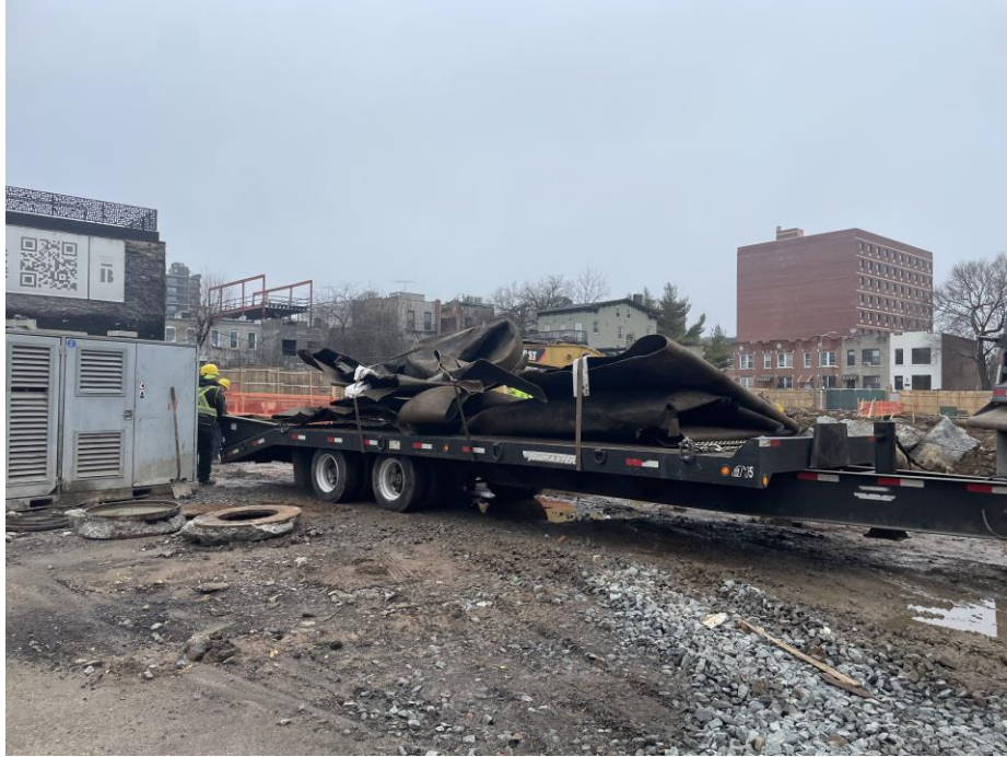
Photo 3: View of Eastern Environmental exporting USTs on Lot 14, facing northeast.
