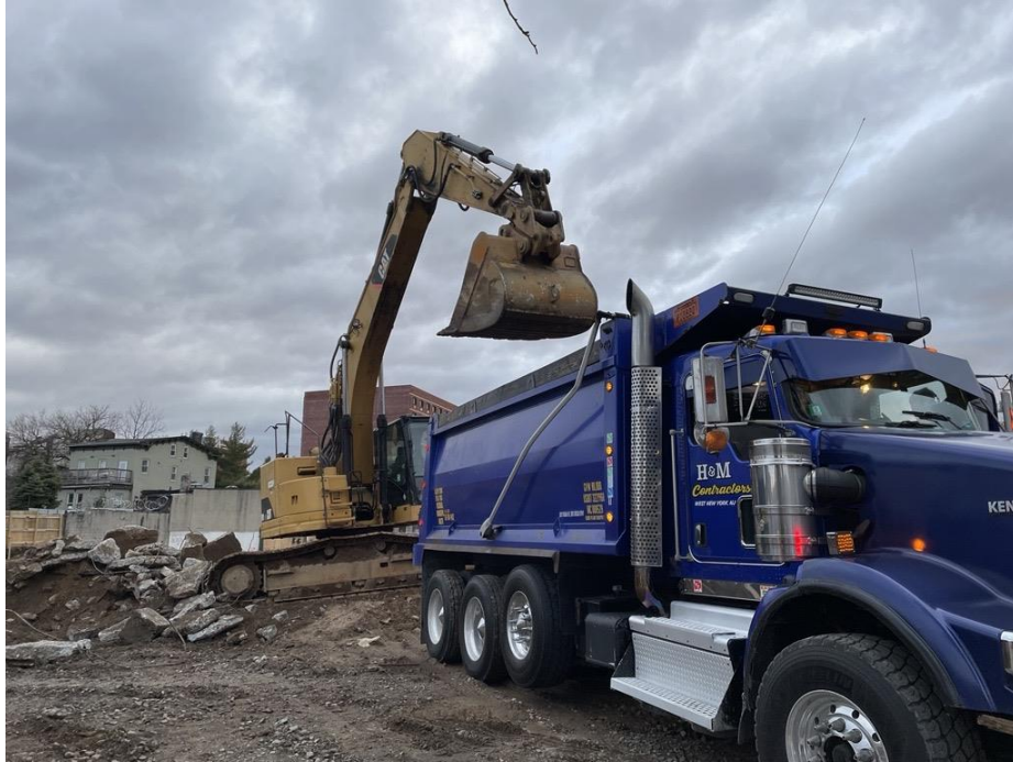
Photo 1: View of C&D disposal in Lot 53, facing east.
