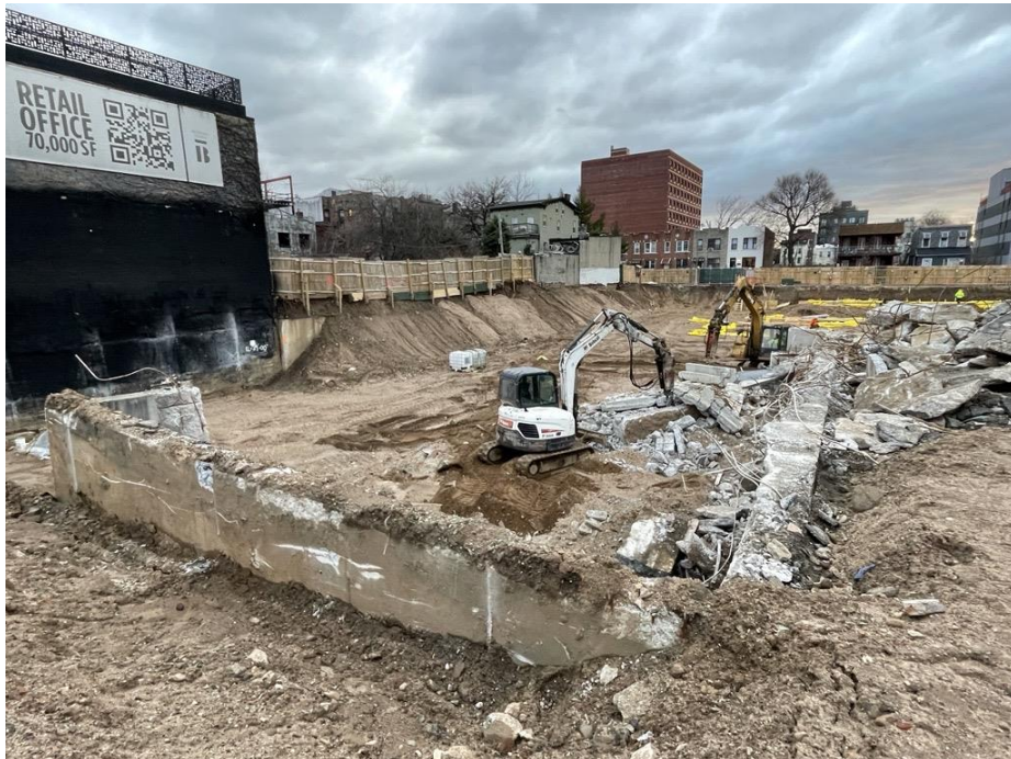
Photo 2: View of concrete demolition in Lot 53, facing east-northeast.
