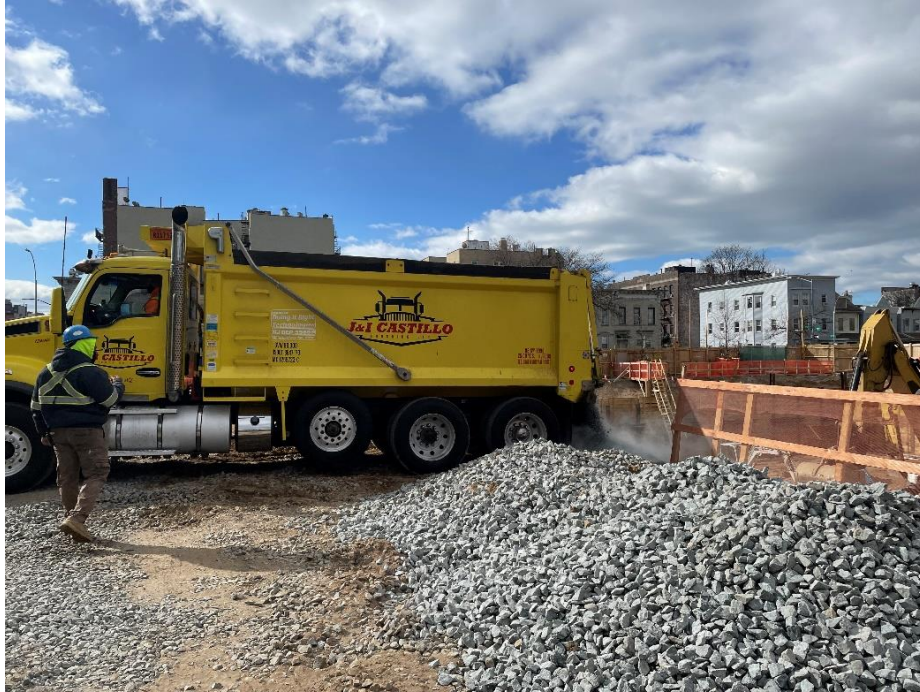
Photo 3: View of clean stone import on Lot 14, facing south.
