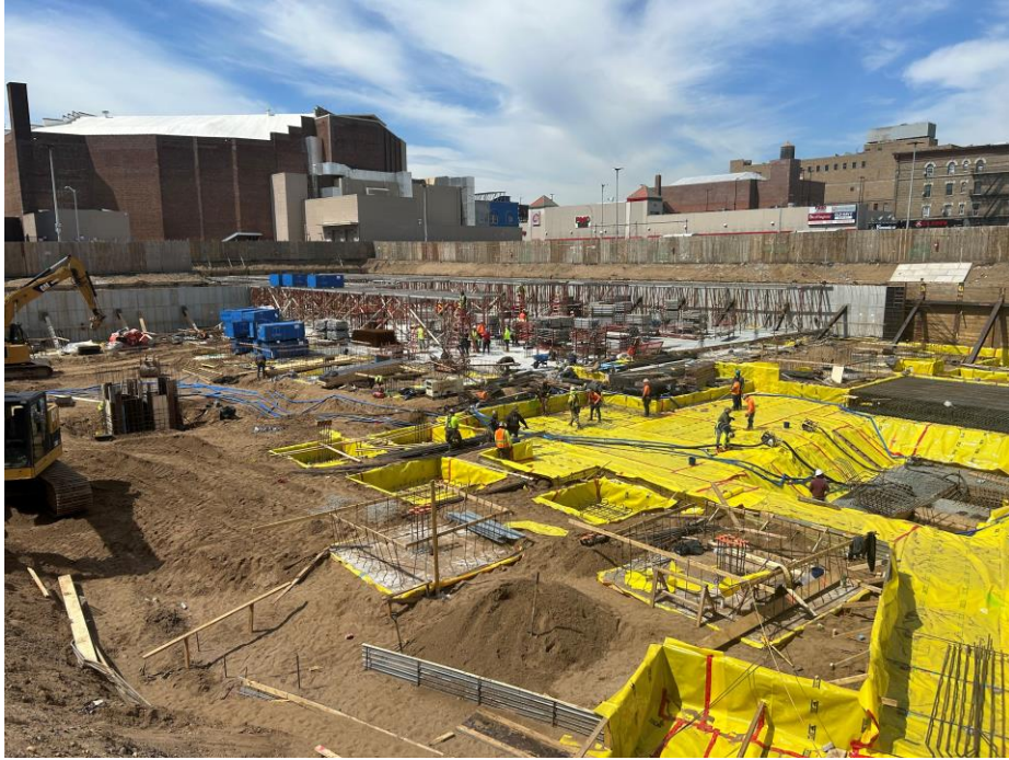
Photo 1: View of site conditions in Lot 14, facing west.
