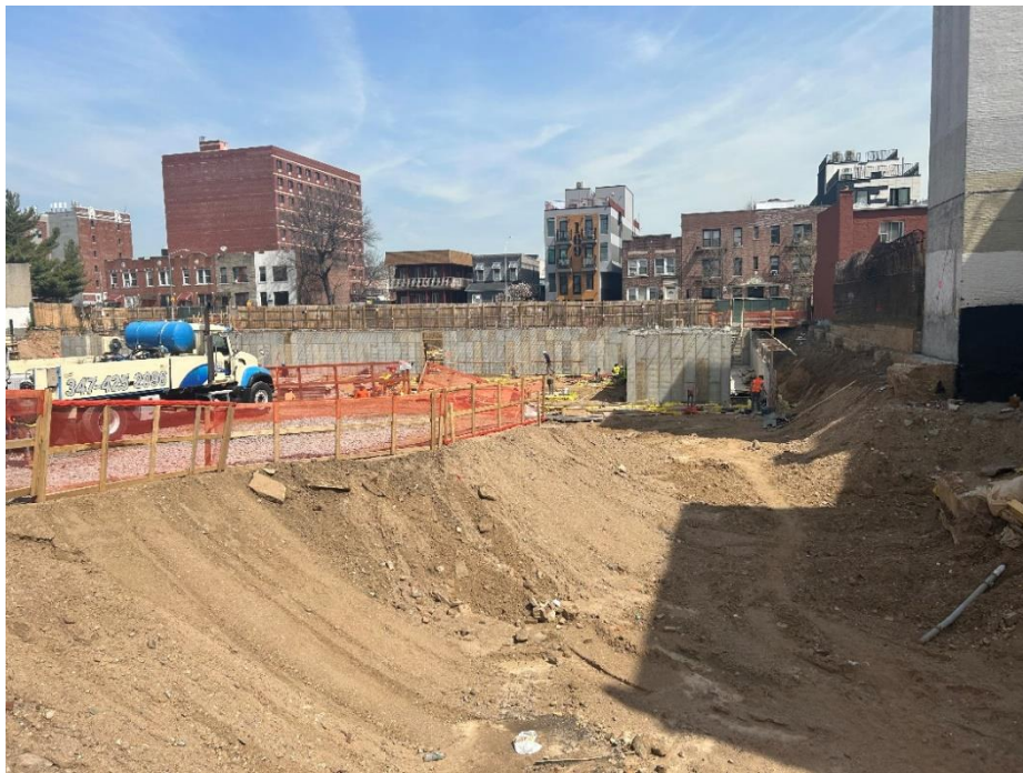
Photo 2: View of site conditions on Lot 53, facing east.
