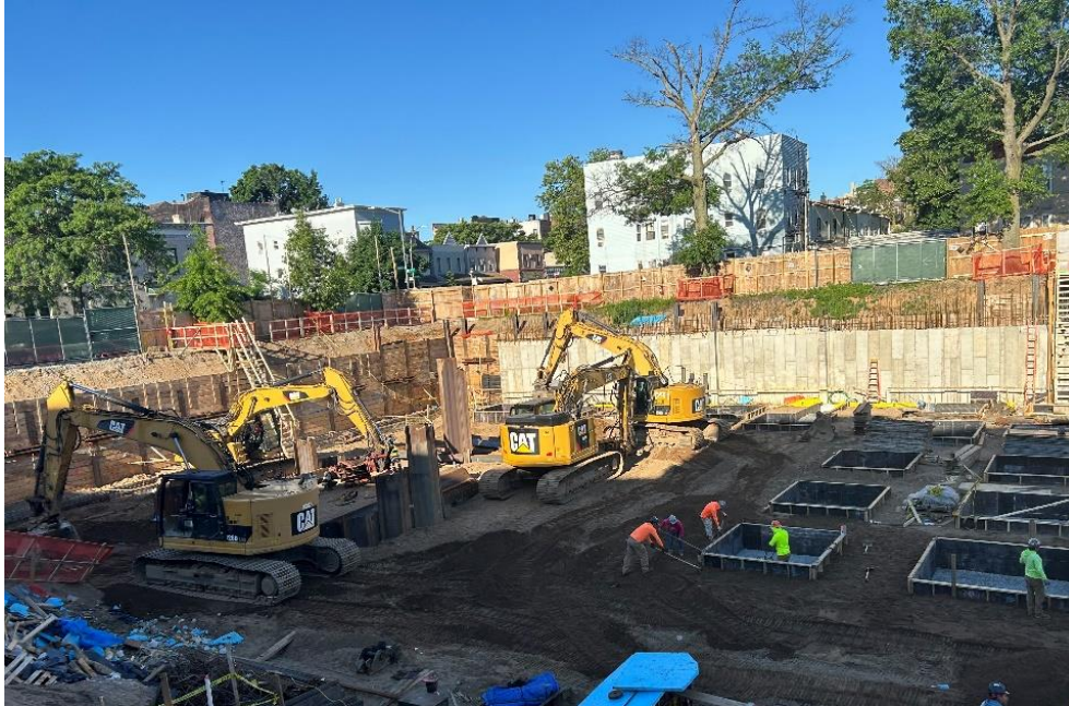
Photo 1: View of site conditions in Lot 14, facing west.
