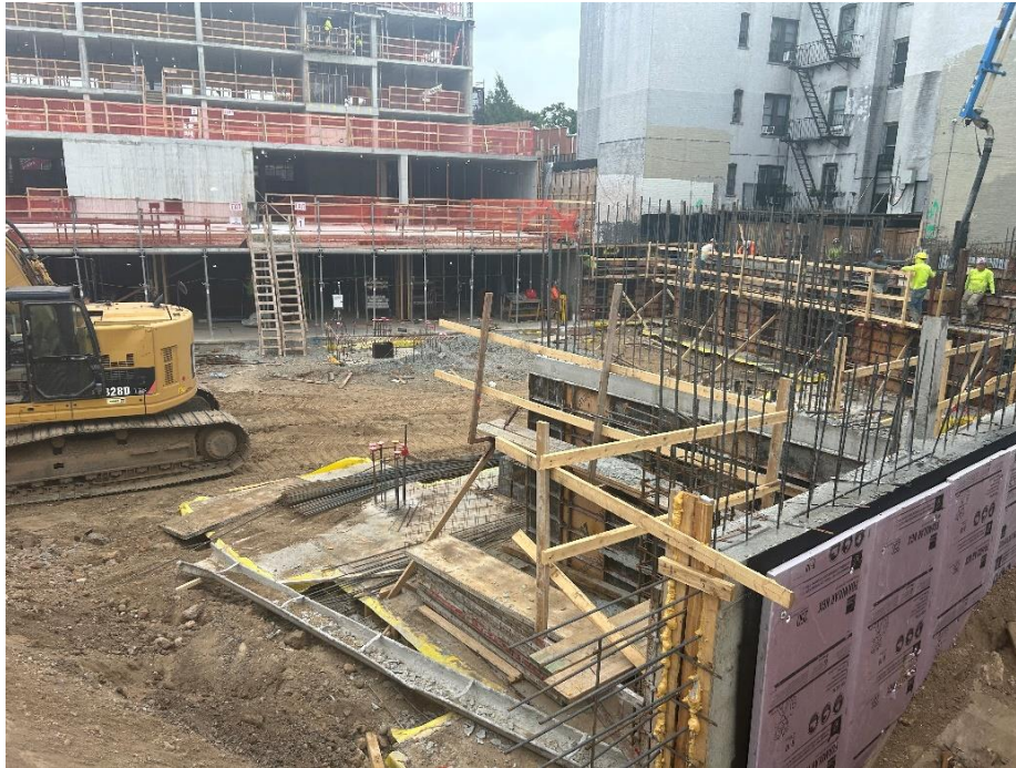
Photo 1: View of site conditions in Lot 53, facing east.
