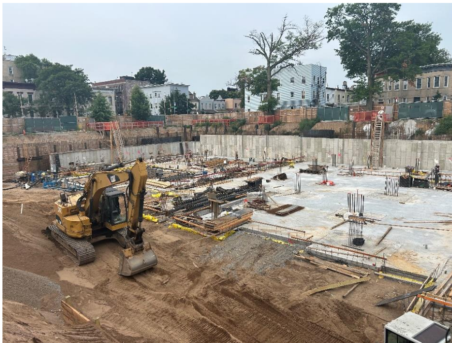
Photo 2: View of site conditions in Lot 14, southwest.
