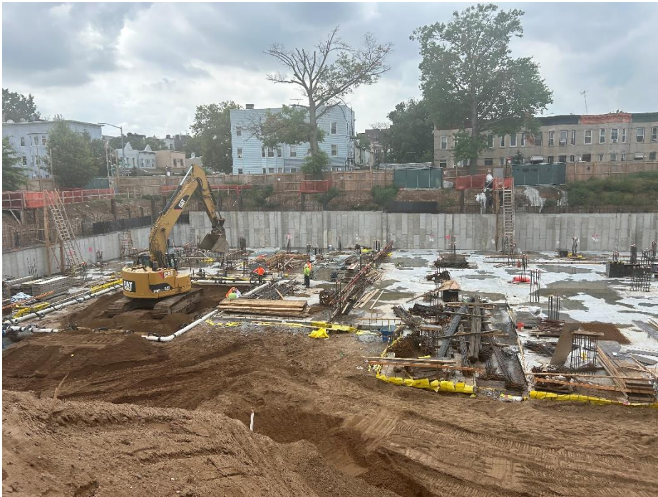
Photo 2: View of site conditions in Lot 14, west.
