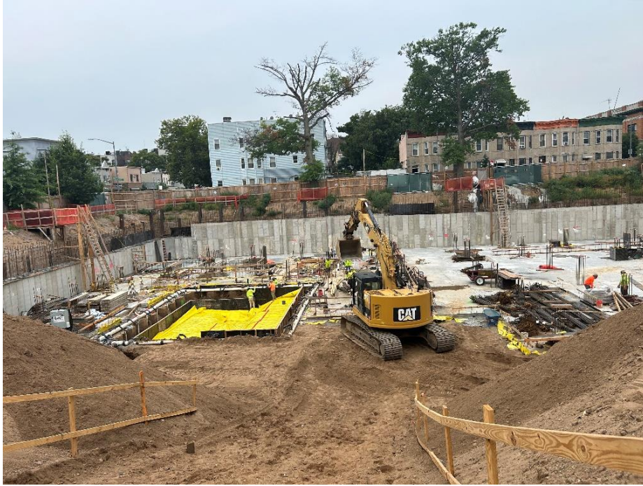
Photo 1: View of elevator pit excavation in Lot 14, facing east.
