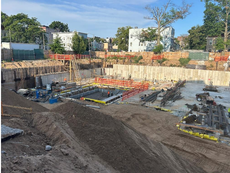
Photo 1: View of elevator pit installation in Lot 14, facing southwest.
