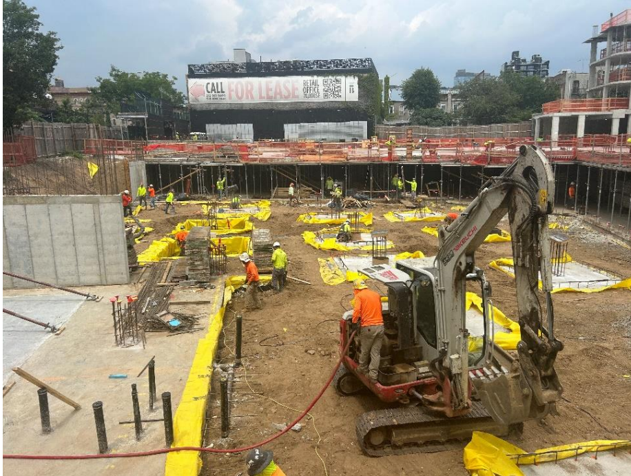
Photo 1: View of footing preparation in Lot 53, facing north.
