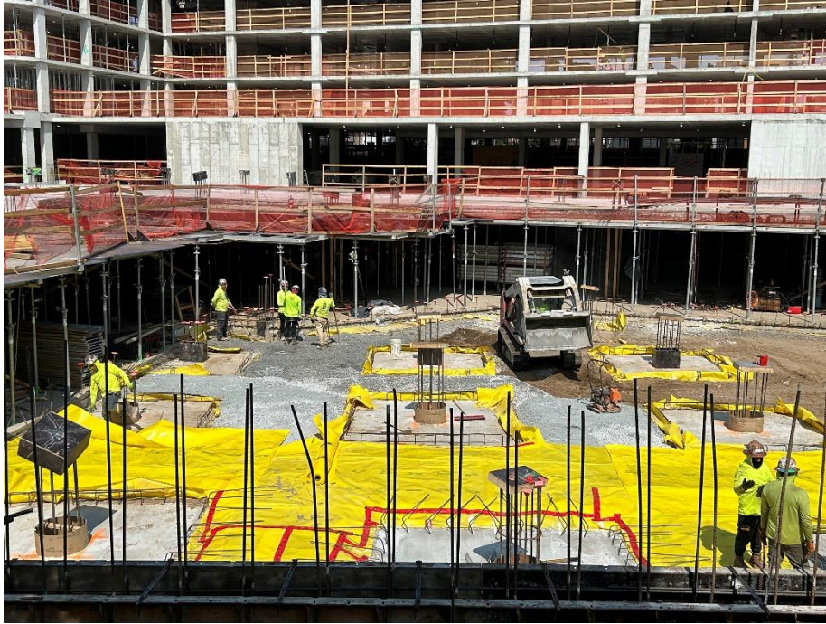
Photo 1: View of footing preparation in Lot 53, facing east.
