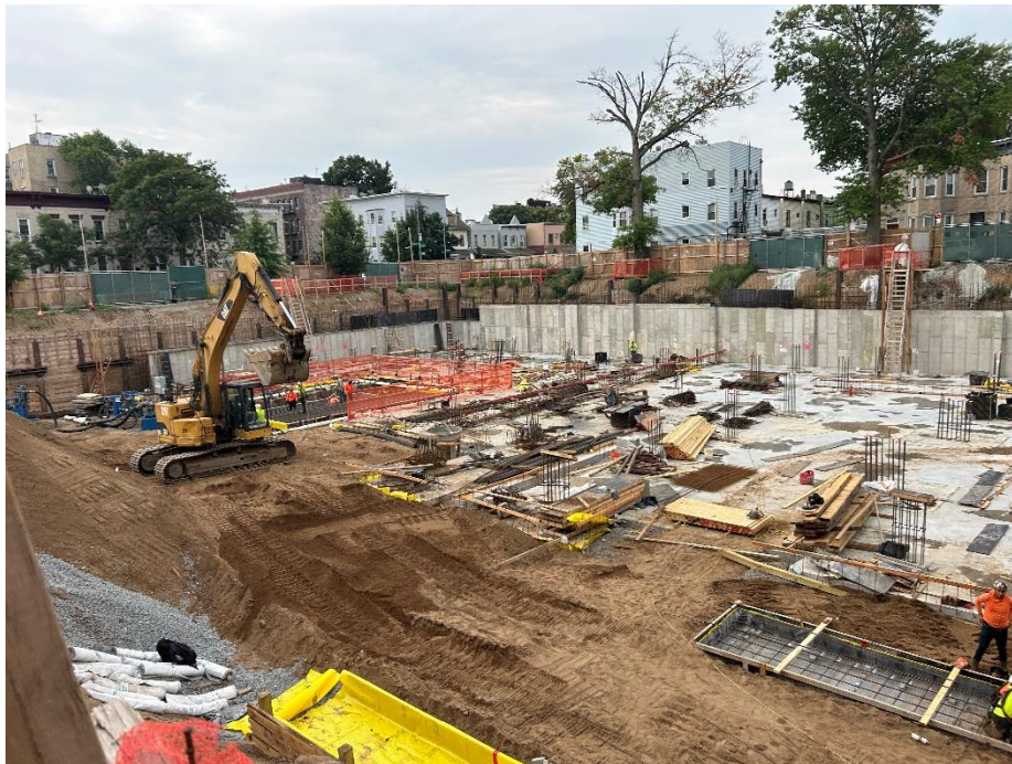
Photo 2: View of site conditions in Lot 14, facing southwest.
