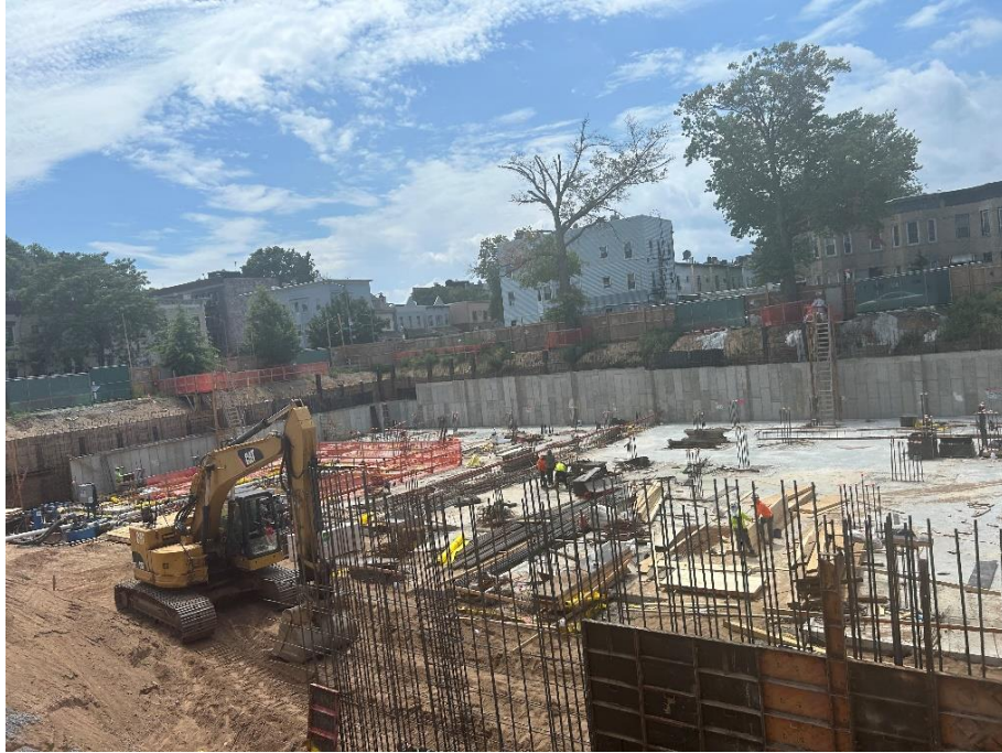
Photo 1: View of site conditions in Lot 14, facing southwest.
