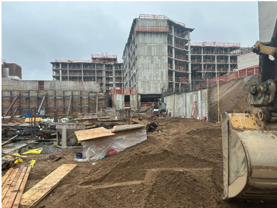
Photo 2: View of site conditions in Lot 14, facing north.
