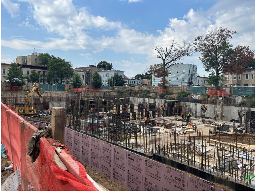
Photo 1: View of site conditions in Lot 14, facing northwest.
