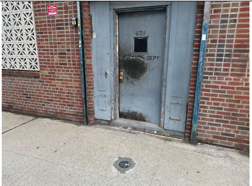
Photo 4: Existing monitoring well (B10D) observed along Union Street.
