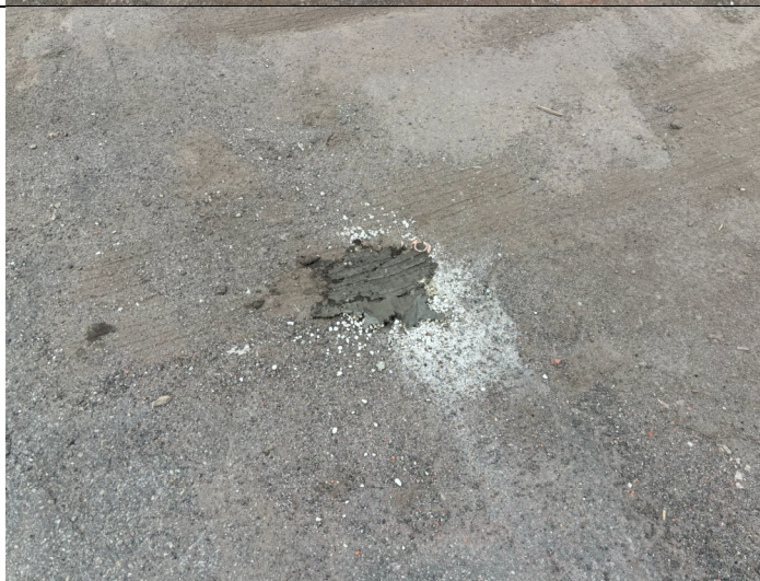
Photo 5: View of decommissioned well 25MW- 7
