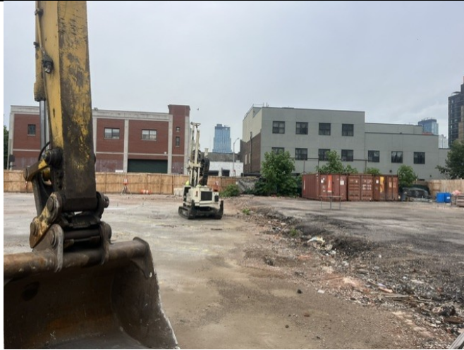
Photo 1: View of installing soil boring 25SB- 4S3 looking north
