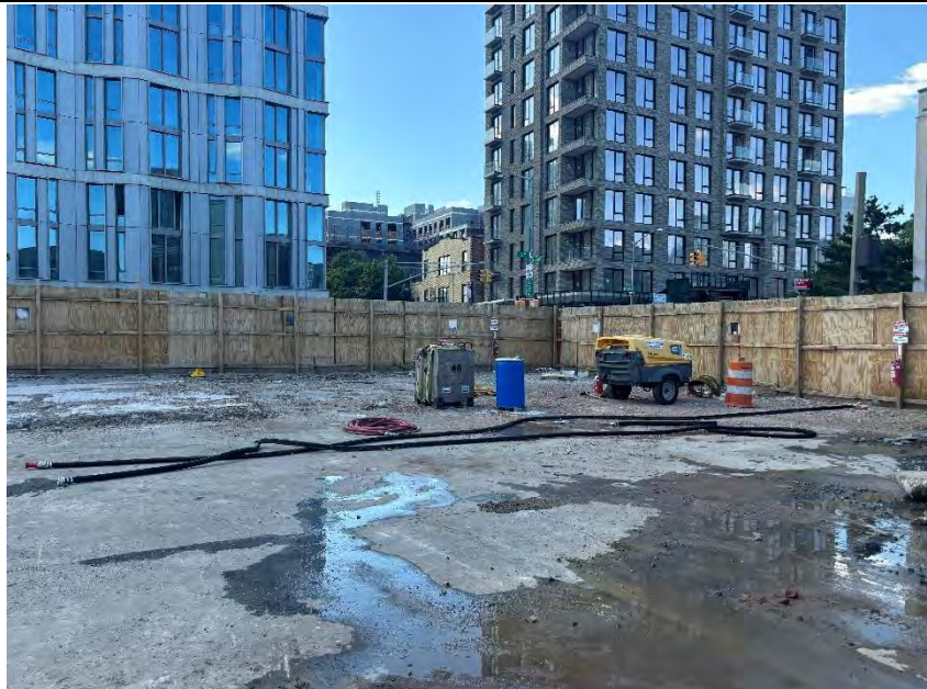
Photo 1: View of atmos foam sprayer and water hose before work starts looking northwest
