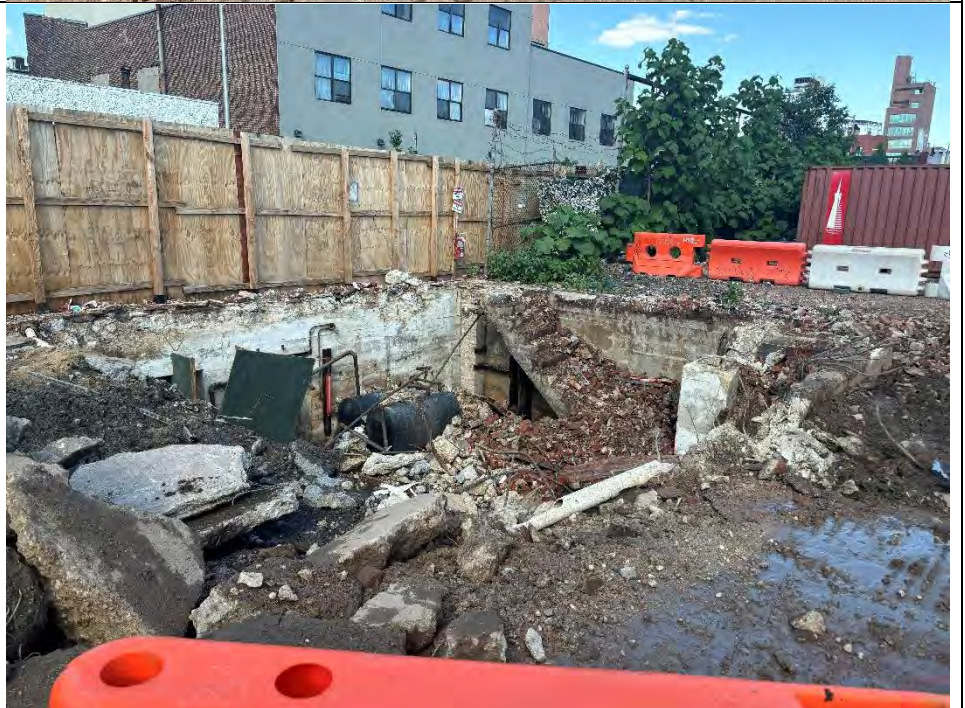
Photo 4: View of the two 275-gallong ASTs facing northeast
