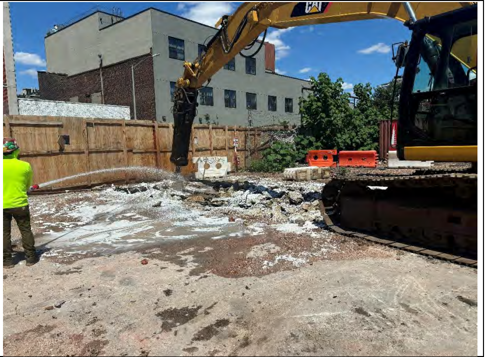
Photo 3: View of atmos foam sprayer tested and water hose use during concrete slab removal looking northeast
