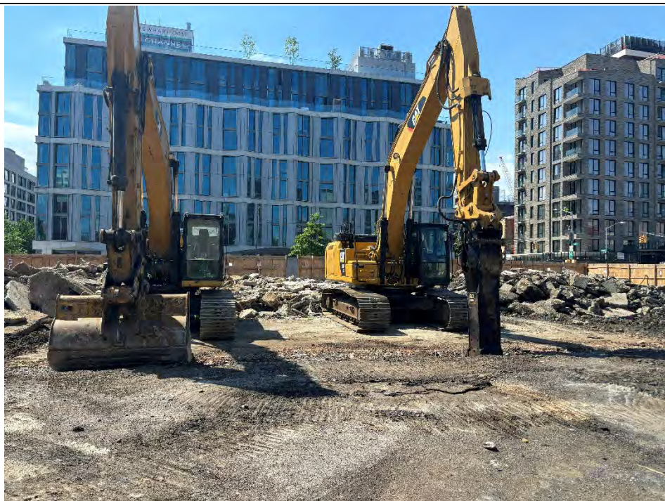
Photo 5: View of idle excavators after the completion of concrete slab removal looking west
