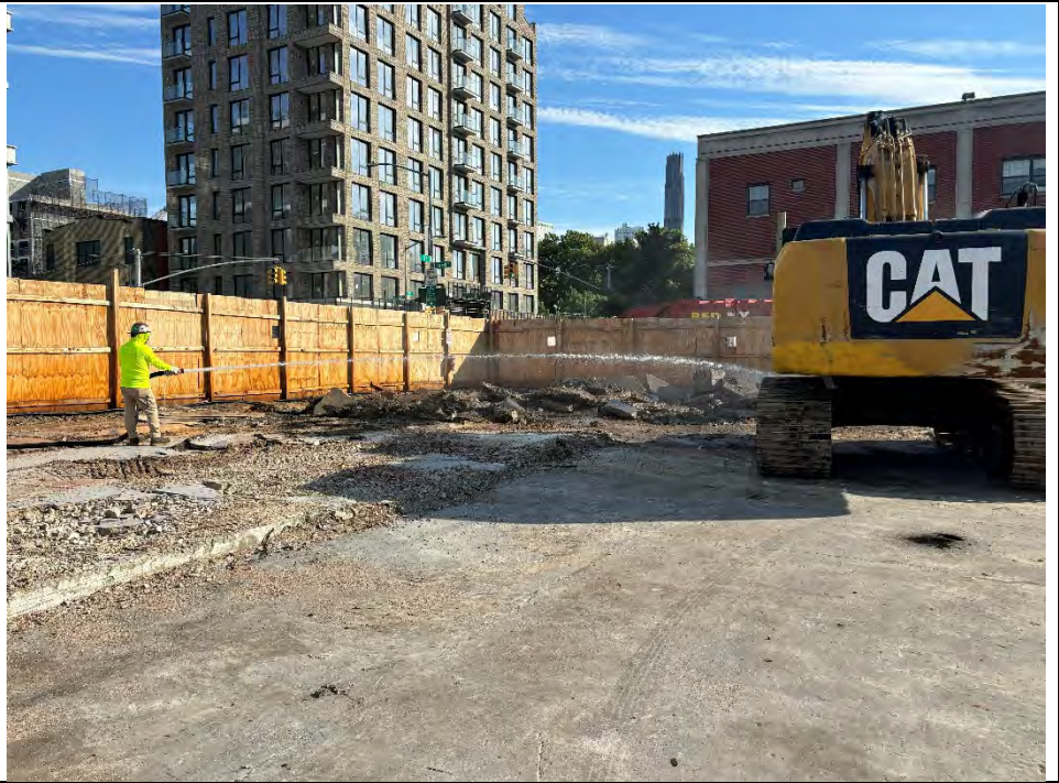
Photo 3: View of water hose use during concrete slab removal looking north
