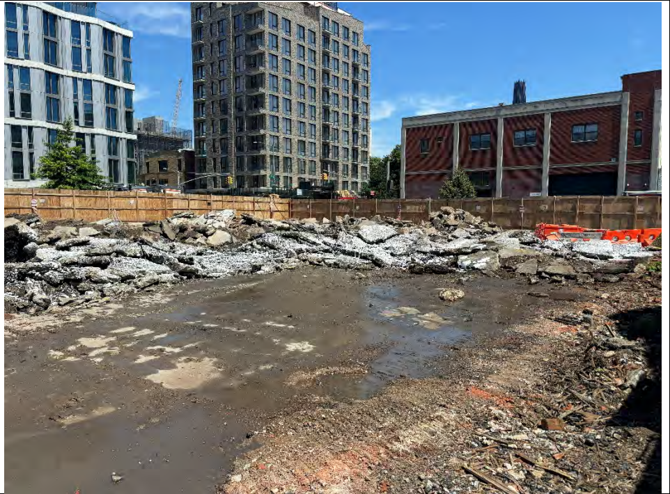
Photo 4: View of partial concrete slab removal with atmos foam use looking northwest
