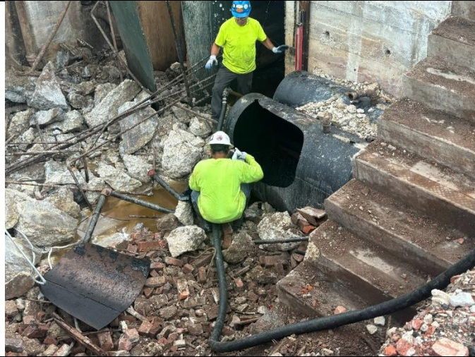
Photo 1: View of cleaning of two 275-gallon ASTs looking northwest
