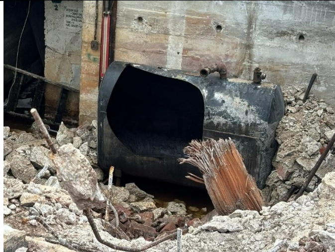
Photo 2: View of extracted 275-gallon AST looking north
