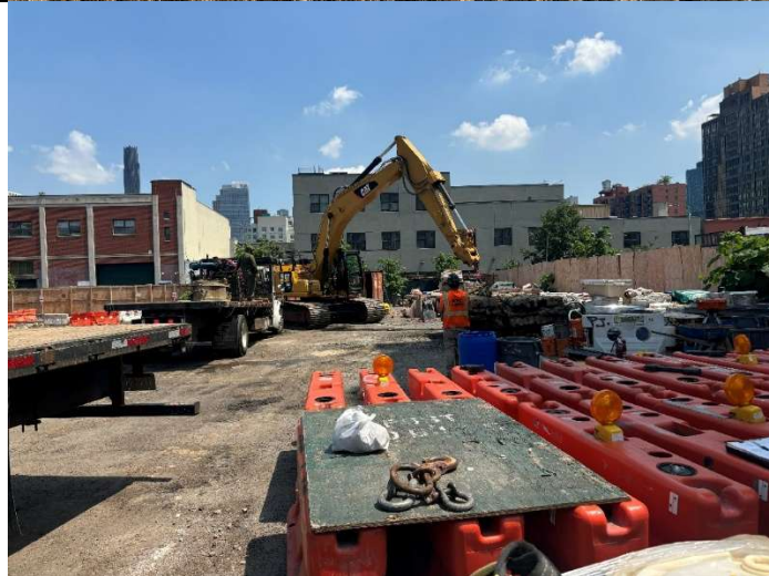
Photo 2: View of wood lagging and drill rig delivery for future SOE looking north
