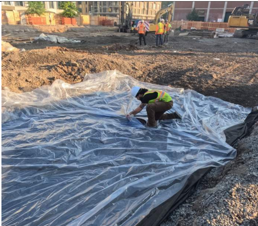
Photo 7: View of trucking pad installation with plastic sheeting being installed over geotextile fabric
