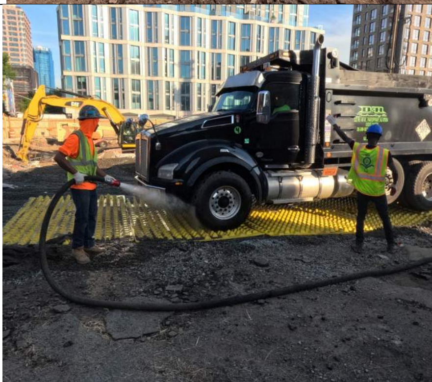
Photo 4: View of the trucking pad and washing area.
