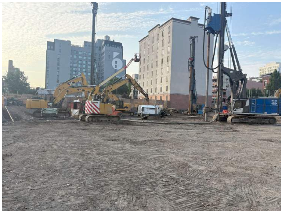
Photo 3: View of the piling activities and site looking east
