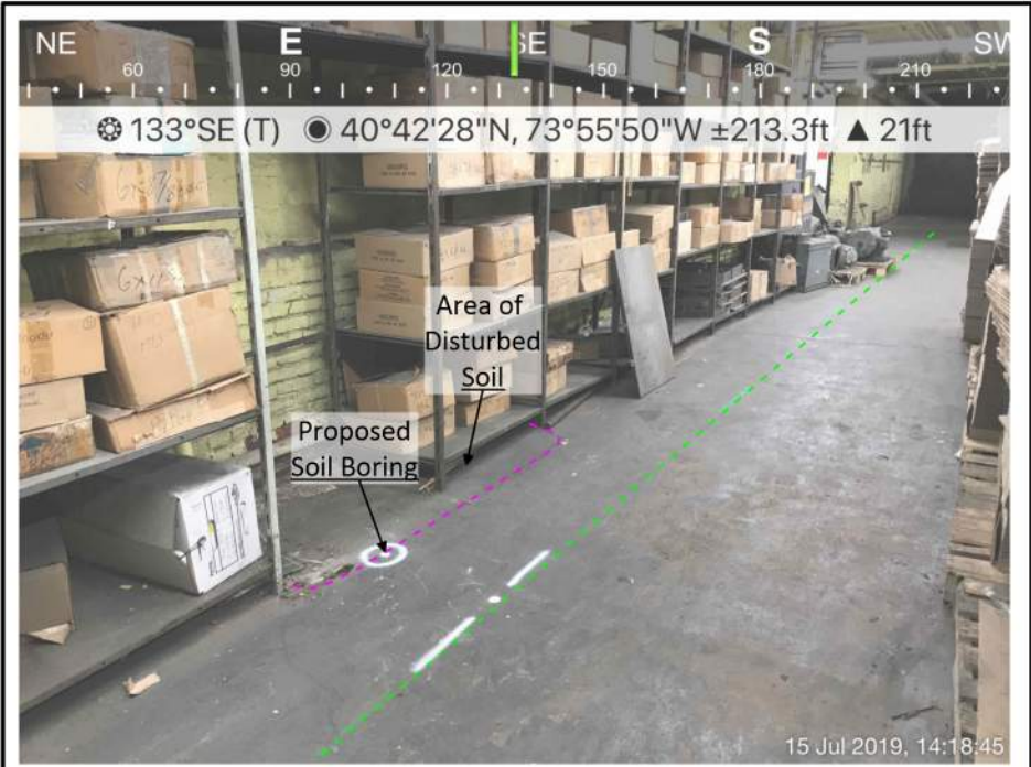
Southeast-looking site photo showing proposed soil boring and detected floor drain. Note that the cut in the concrete is present where two suspected supply/return lines terminate. SET observed disturbed soils in the indicated area (dashed-magenta).
