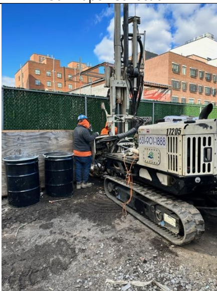
Soil Vapor Probe Installation
