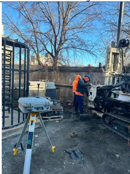
CAMP Station and Soil Probe Installation
