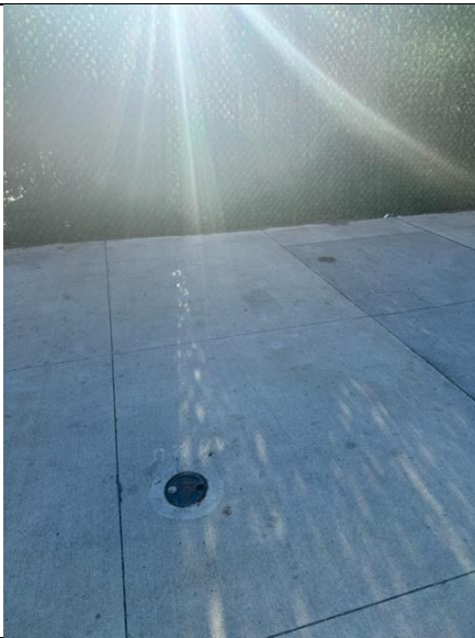
Exterior Monitoring Wells
