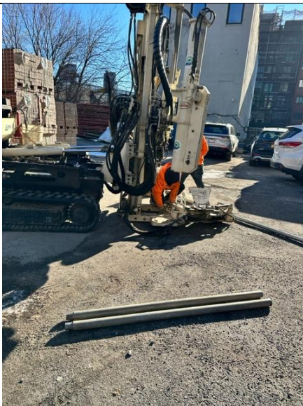
Soil Probe Installation
