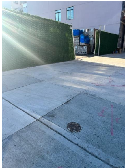
Exterior Monitoring Wells
