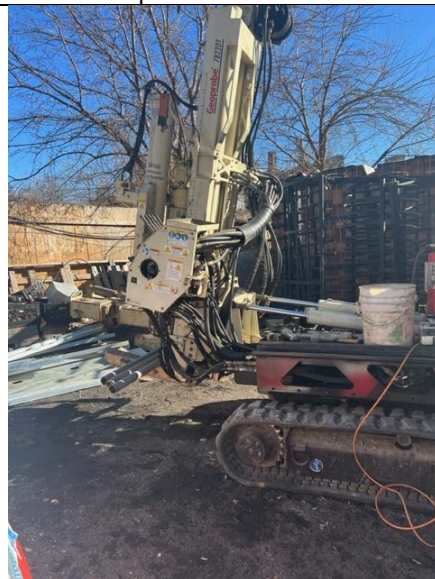
Soil Probe Installation
