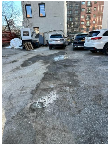
Soil Vapor Probe Installation
