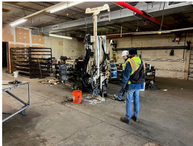
Photo 5. Drilling at SB-2/TMW-2 in the center of the Building.
