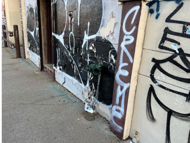
Photo 1. Location of OA-1 on the southeast corner of the Building.
