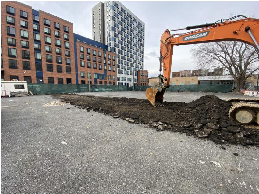
Photo 1: View of Precise removing asphalt in the southwestern part of the site (facing northwest).
