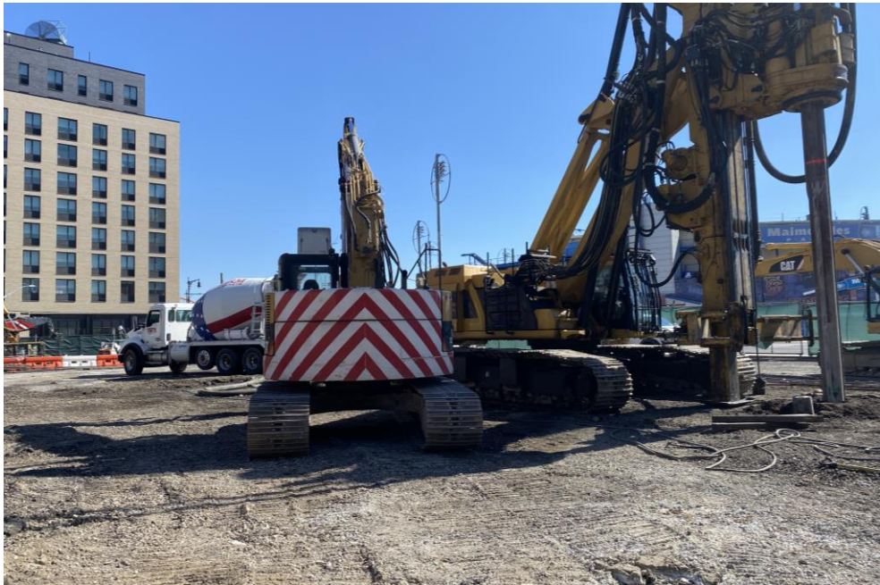
Photo 1: RYC Turbos Corp. installing a pile in the southern part of the site (facing southeast).
