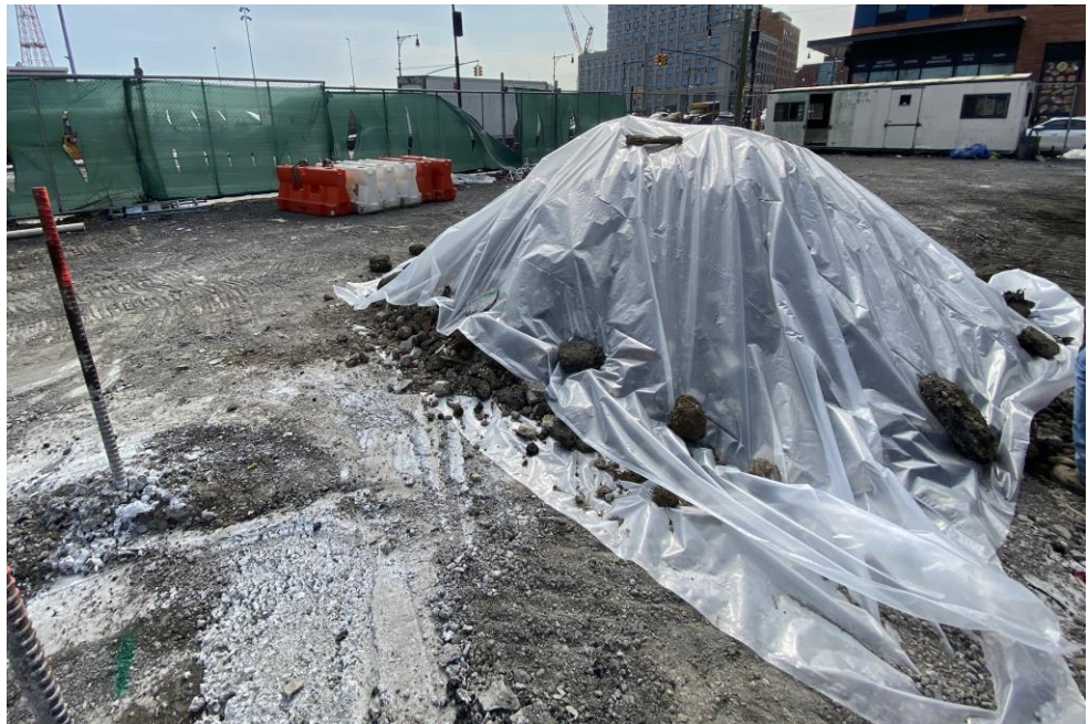
Photo 2: View of stockpiled non-hazardous fill/soil covered with polyethylene sheeting at the end of the work day (facing southwest).
