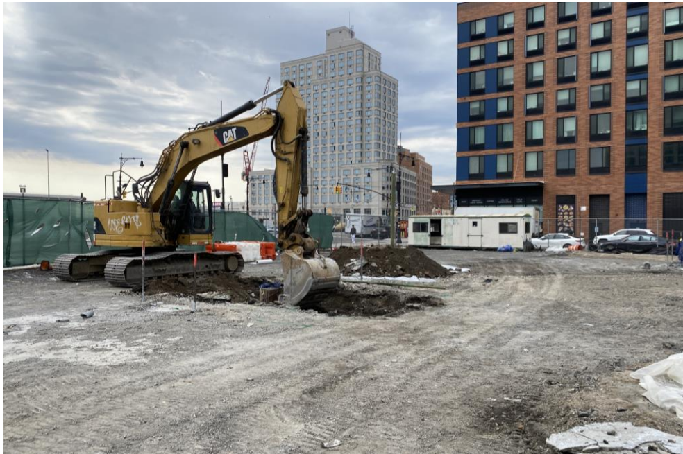
Photo 1: View of RYC Turbos Corp. excavating non-hazardous fill/soil in the southern part of the site (facing southwest).
