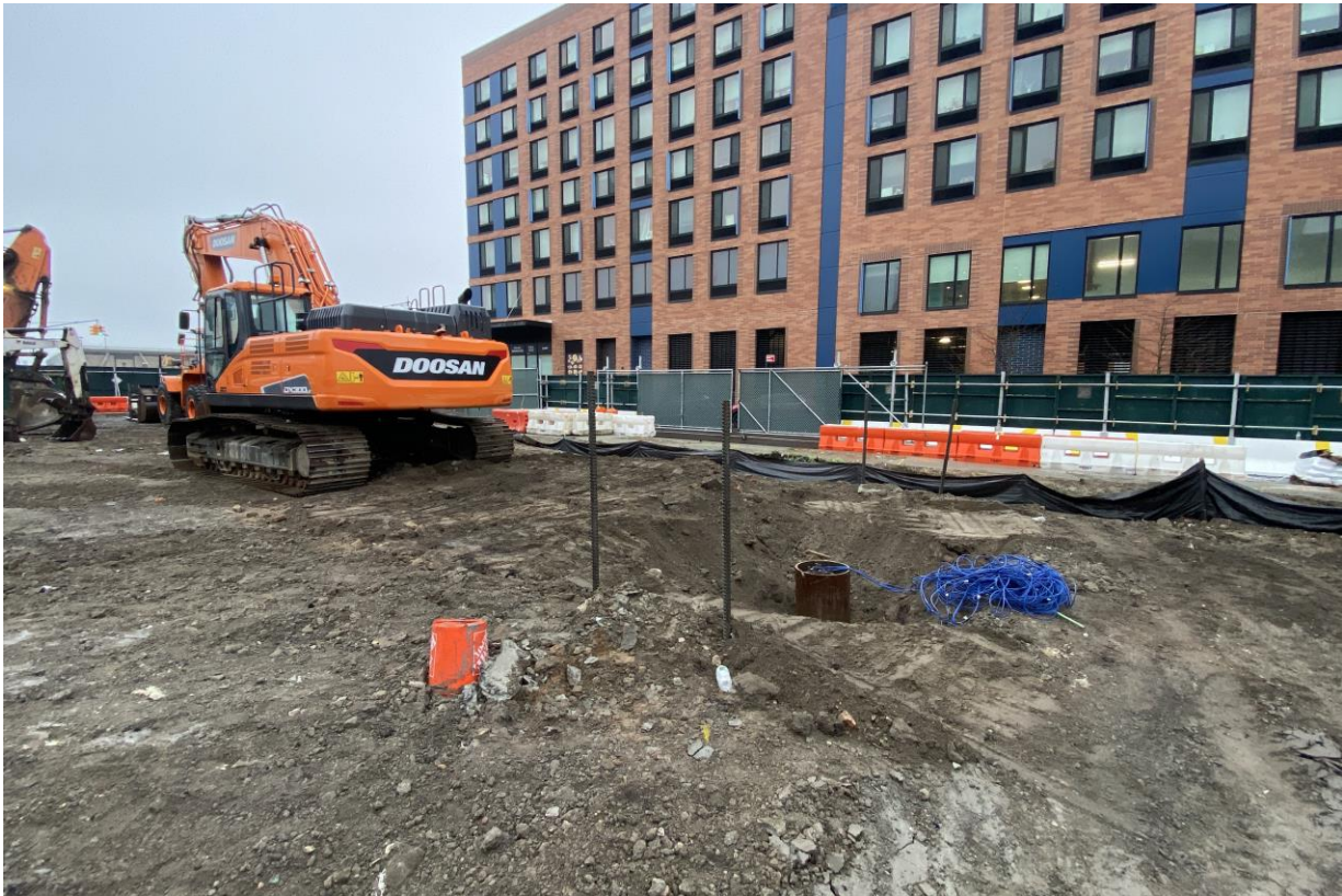
Photo 1: Excavation to support pile test in the western part of the site (facing southwest).
